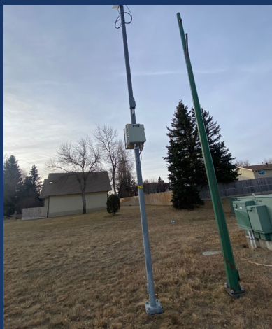
CTM-ONE inside a gatekeeper enclosure, pole-mounted
