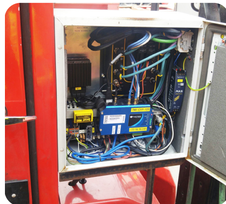
Image 2: CTM-200 device installed in one of Termont's forklift electrical control boxes
